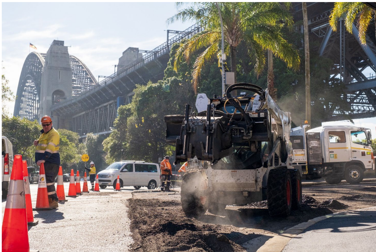
Image 3. Road resurfacing works on Cumberland Street, The Rocks in July 2024. Chris Southwood/City of Sydney
